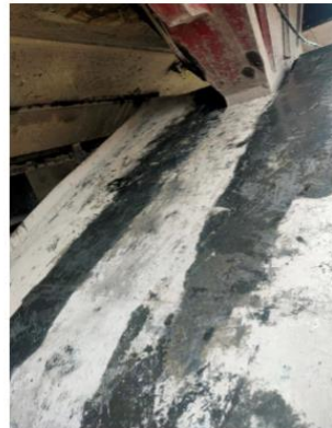
Shoes after bulk grease removal. All surface bulk grease removed. Job completed.
