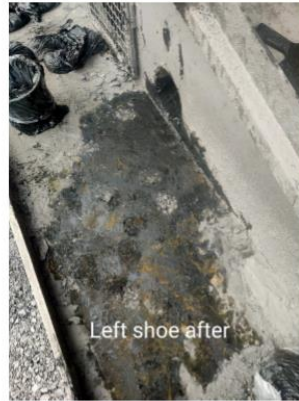
Shoes after bulk grease removal. All surface bulk grease removed. Job completed.
