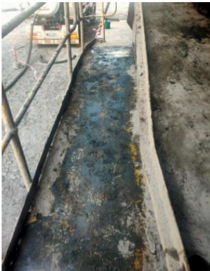
Shoes after bulk grease removal. All surface bulk grease removed. Job completed.
