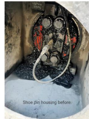
Shoe pin housing before and after bulk grease removal. Job completed.
