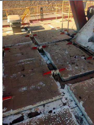
e. Secure/Remove loose items not required on house roof and walkways
