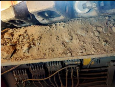
p. Clean and remove dirt, rocks, and debris from tracks
