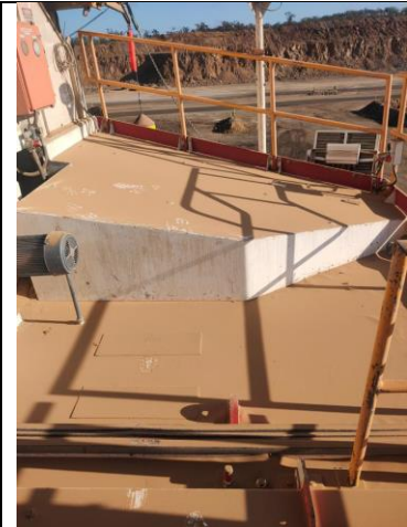
d. Clean House Roof (Deck, Drains and Handrails)
