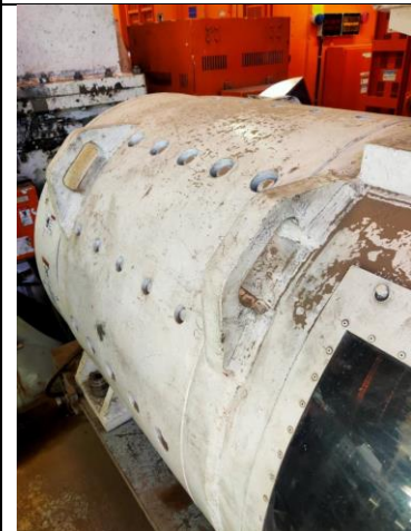
i. Remove dust from motor
