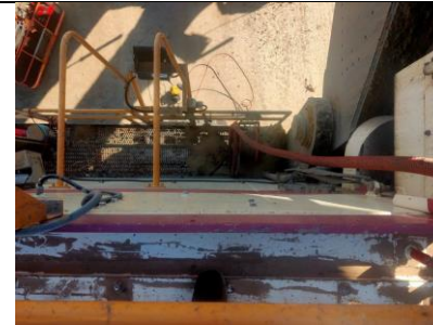
r. Clean out of walkway area in front of the machine
